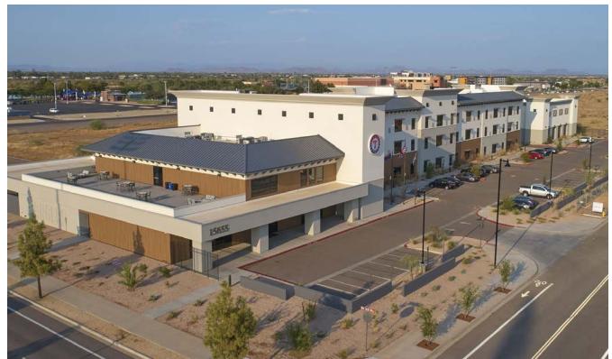
Texas Rangers Housing Facility Construction, Surprise, AZ | GCON
