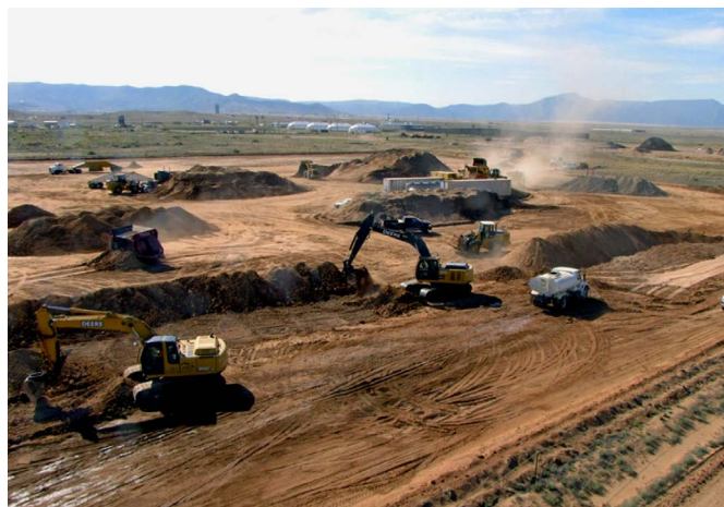
Mixed Waste Landfill and Evapotranspirative Covers Project, Sandia National Laboratories.
